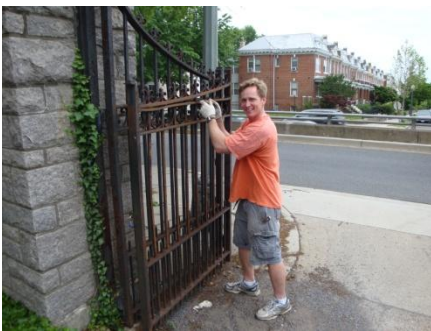
Preparing front gate for new paint
