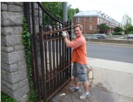
Preparing front gate for new paint
