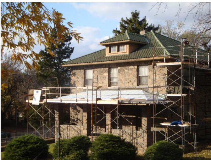
Tiles removed from front porch and new underlayment installed
